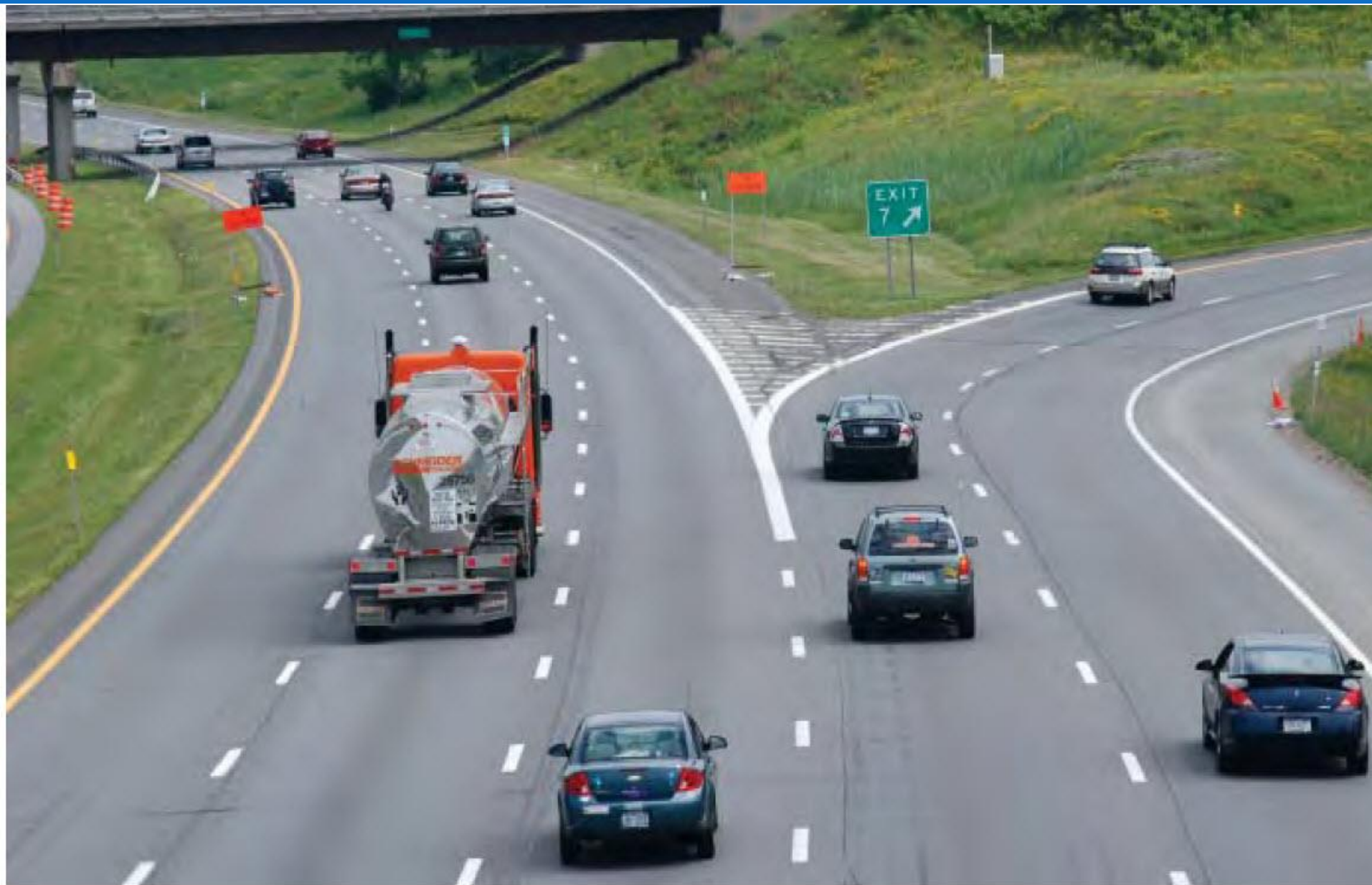
Figure 10-66. Gore Area, Two-Lane Exit
