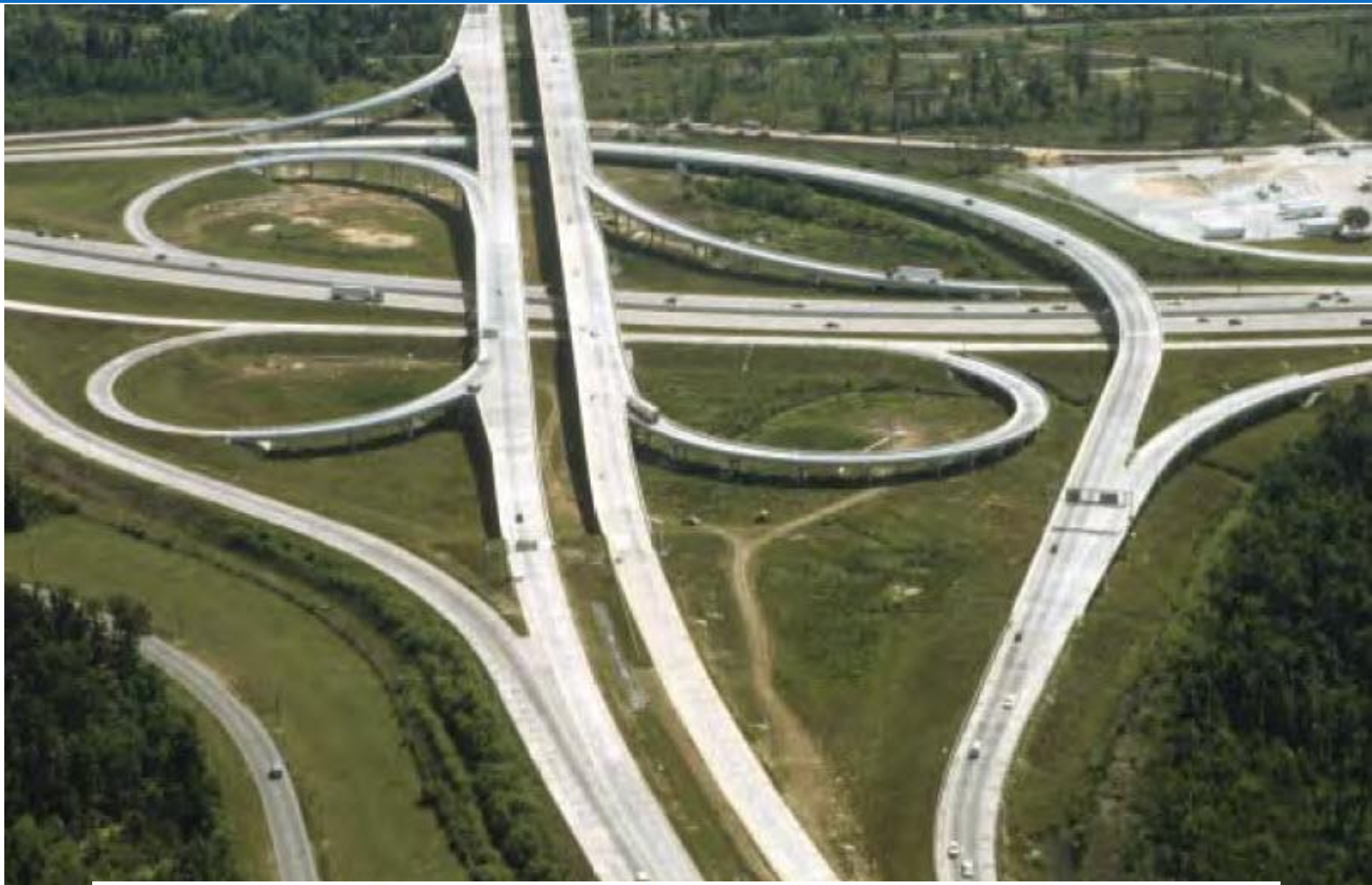
Figure 10-42. Cloverleaf Interchange with Semidirect Connection
