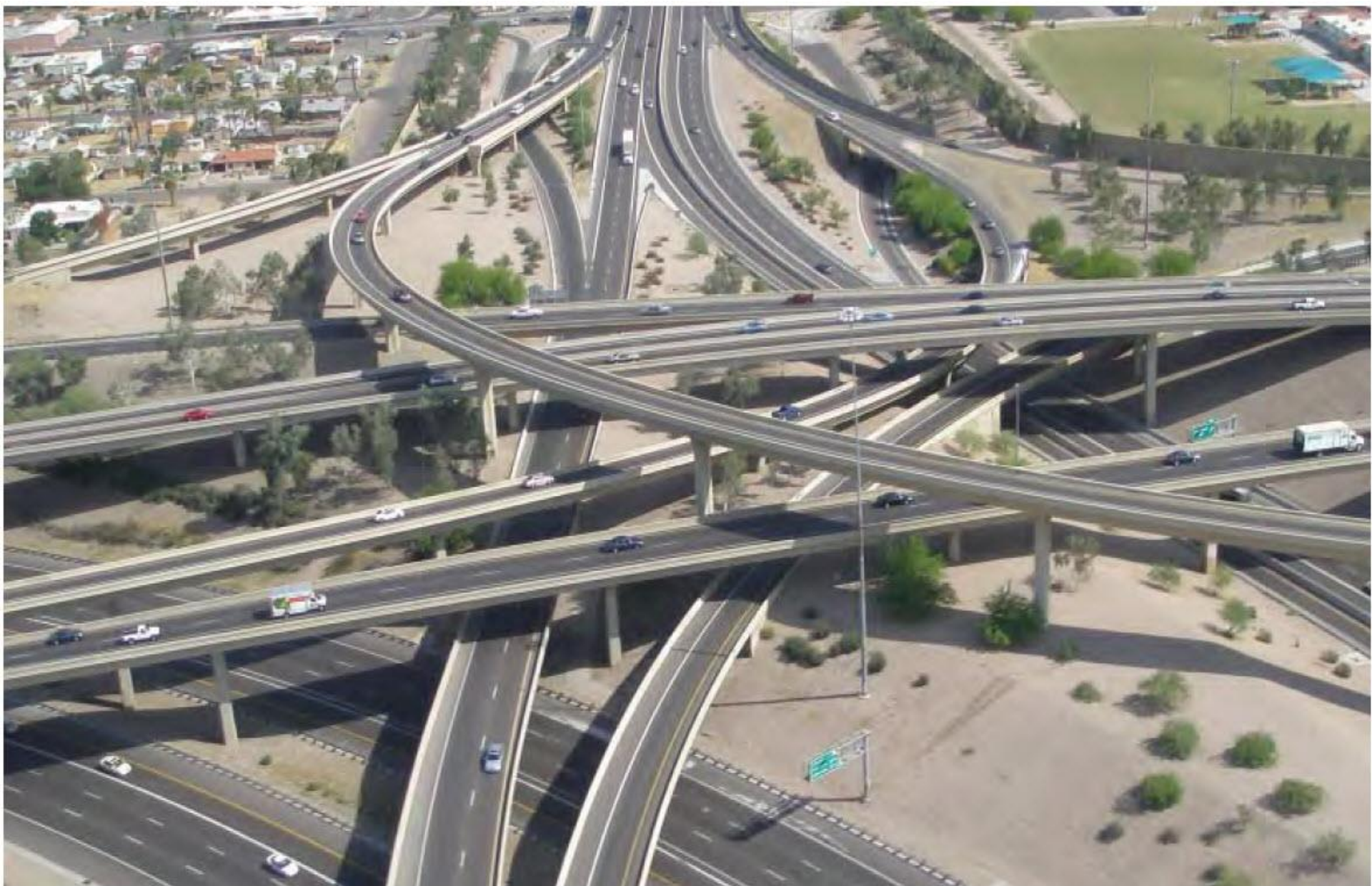
Figure 10-37. Four-Level Directional Interchange
