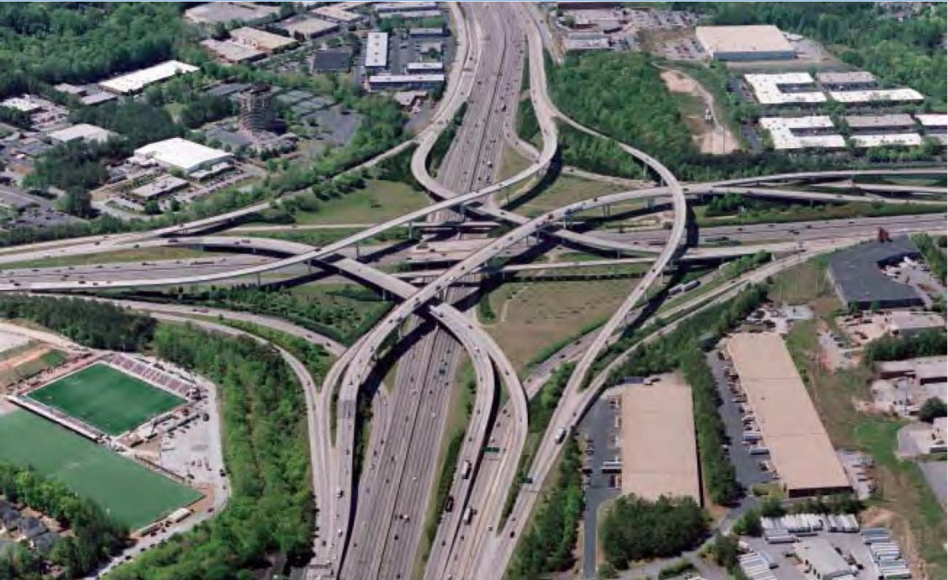
Figure 10-36. Four-Level Directional Interchange
