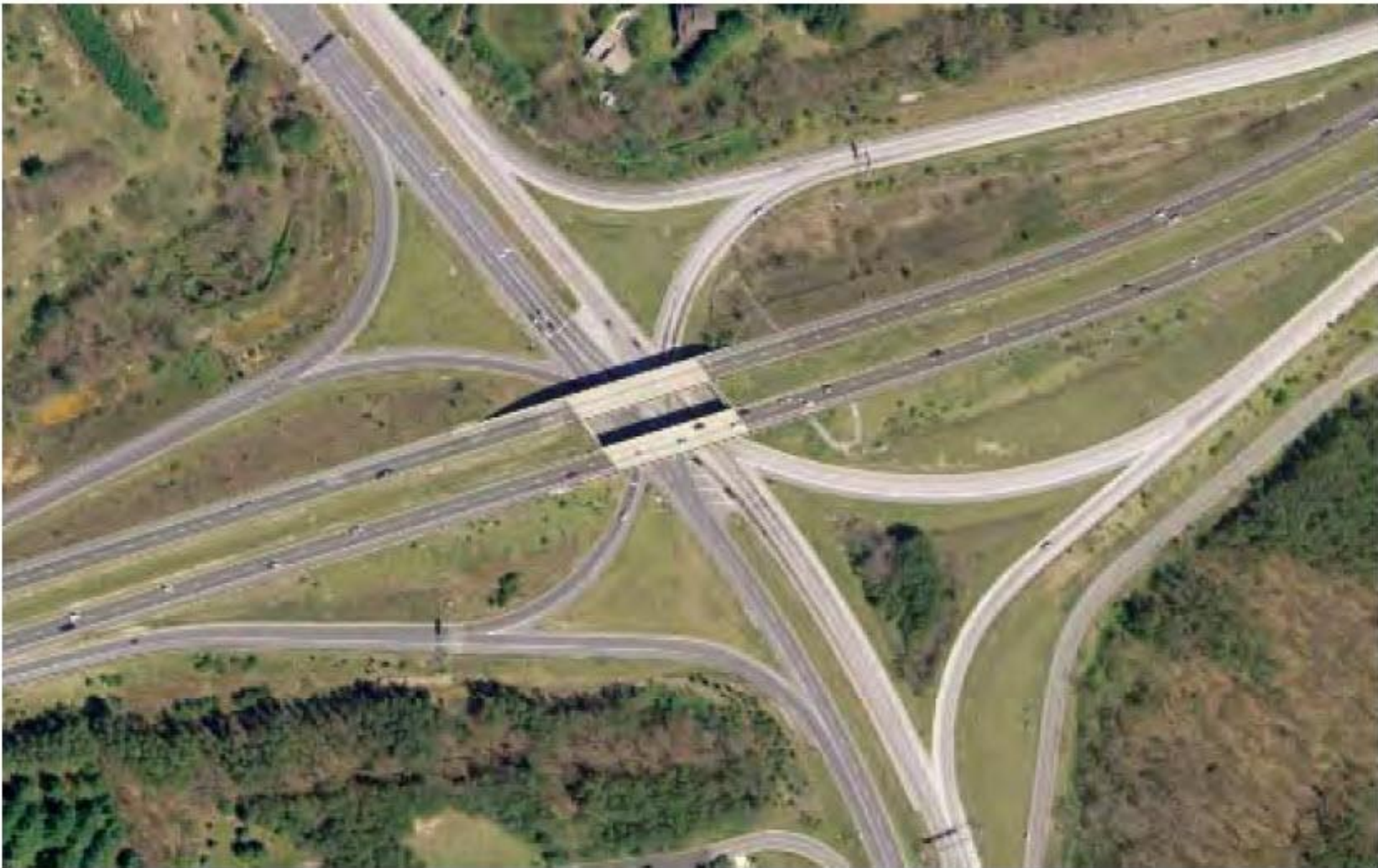
– B – Overpass SPDI
