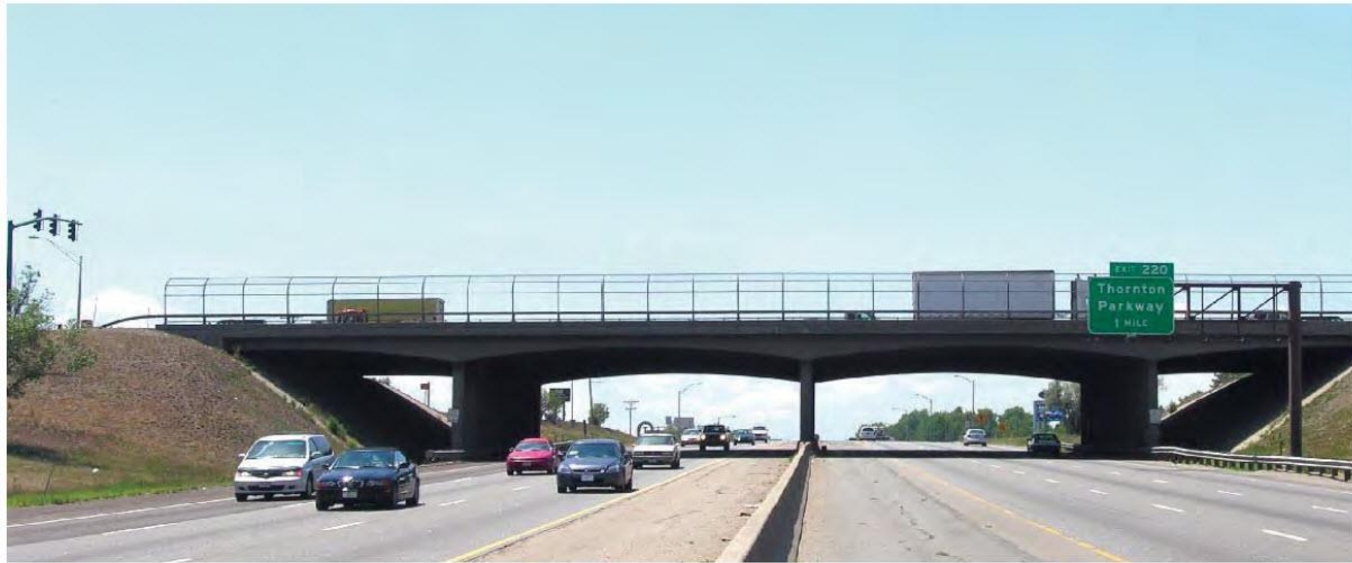
Figure 10-4. Typical Grade Separation Structure with Open-End Span
