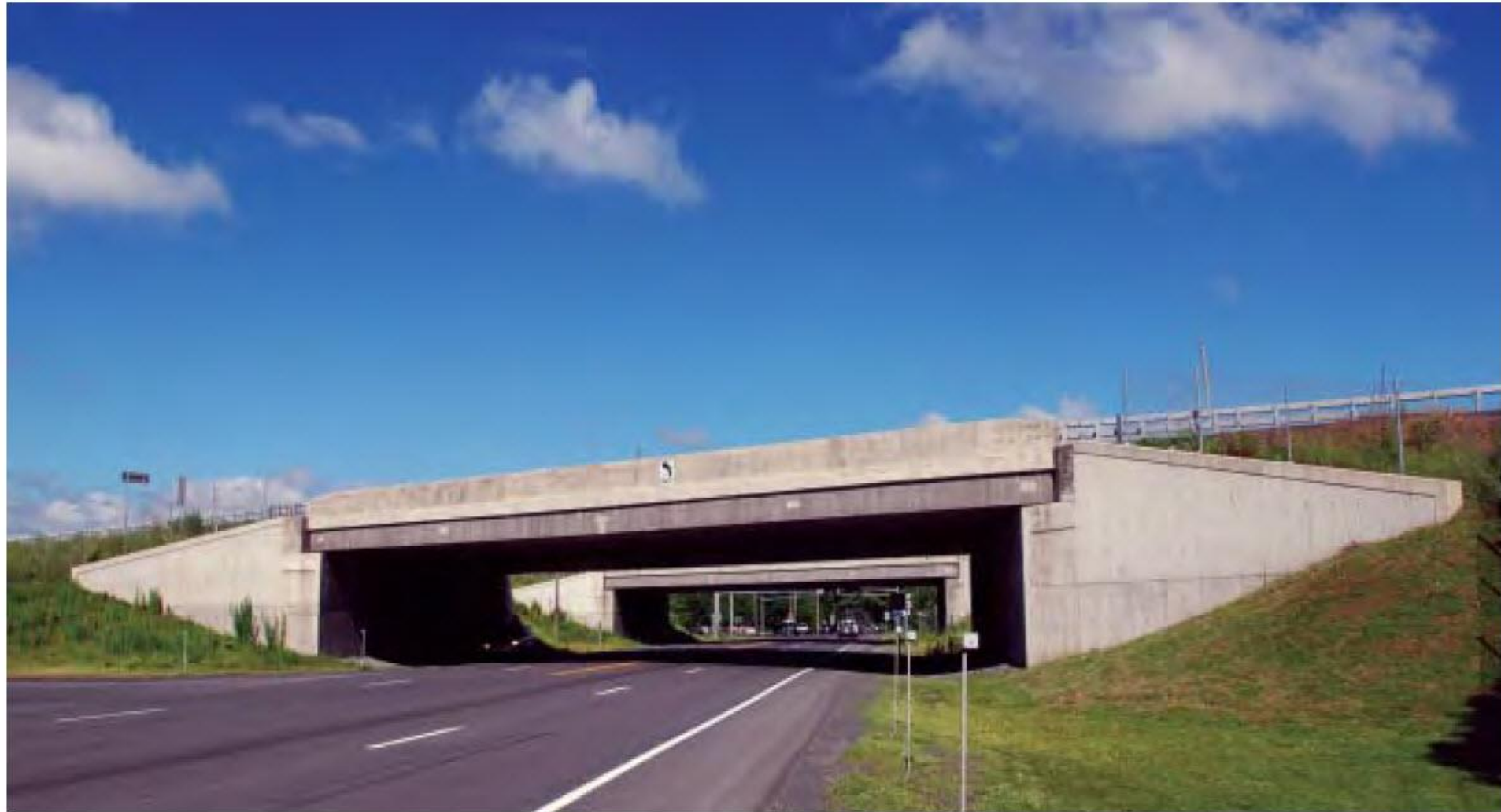
Figure 10-3b. Typical Grade Separation Structures with Closed Abutments
