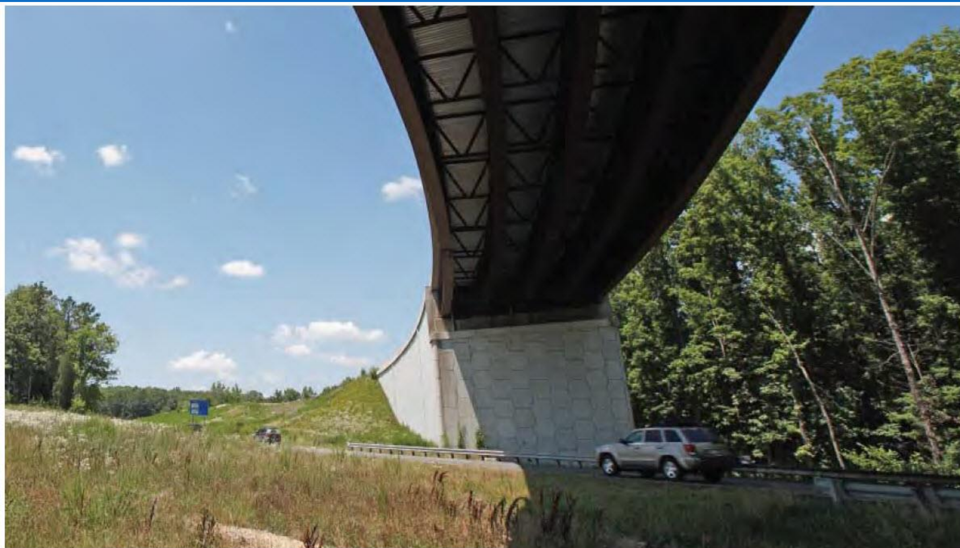
Figure 10-3a. Typical Grade Separation Structures with Closed Abutments
