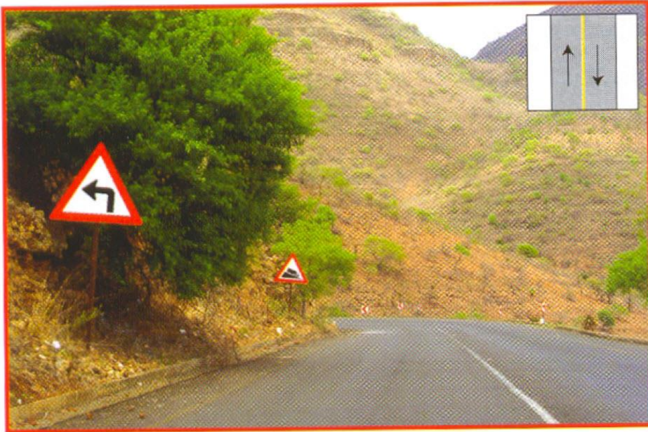
Combination of a downhill grade and sharp horizontal curve creating a sight distance restriction
